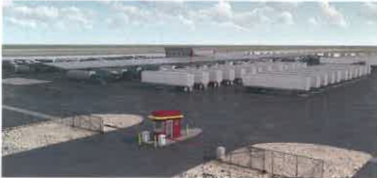
Site Entry at East Barbour Street
