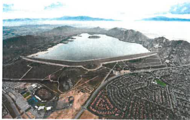
An aerial view of Lake Perris and Perris Dam. Source: DWR
