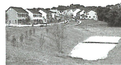
Sand filter at the base of the bioswale promotes infiltration.
