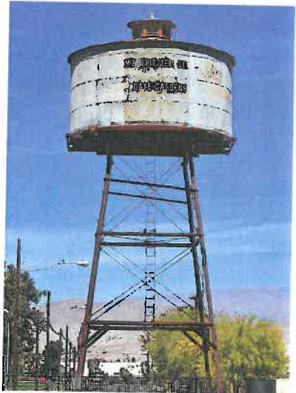
Indio's water tower at the Date Museum
