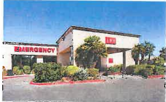
JFK Memorial Hospital Indio, CA
