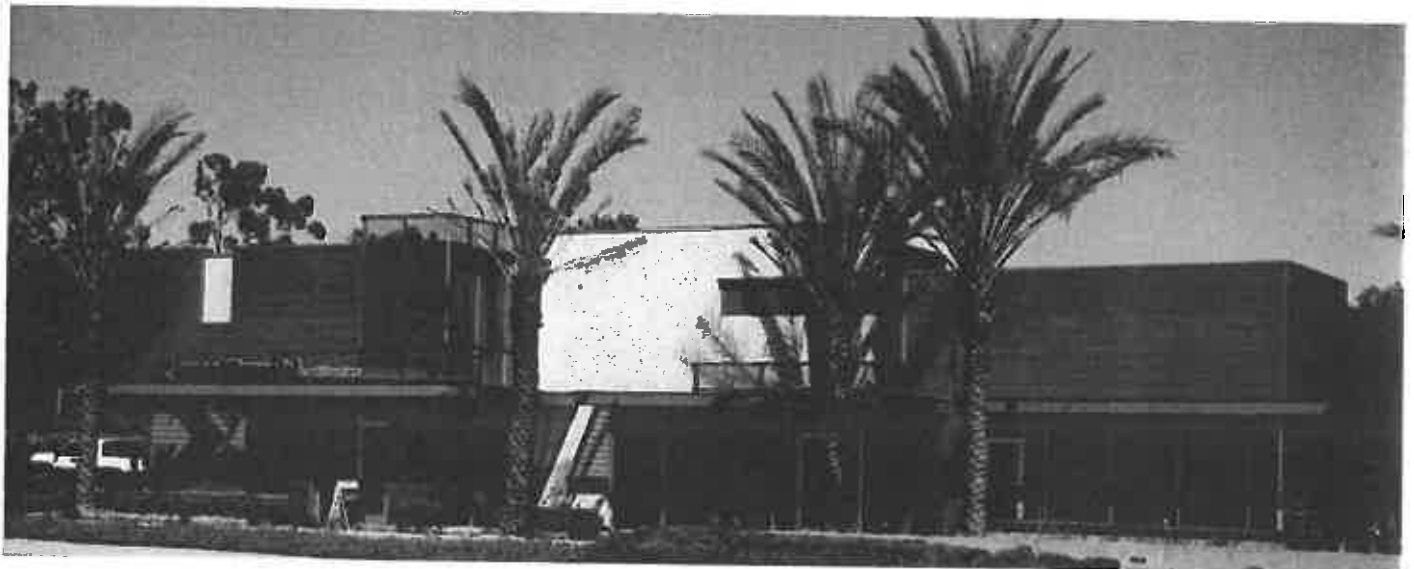
Facade materials blended for walls and roof screens
