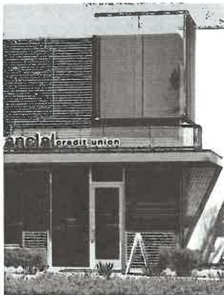
Metal siding with accent screen panels
