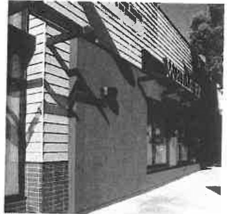
Horizontal siding with stucco
