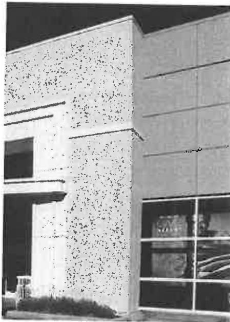
Exposed integral color concrete
