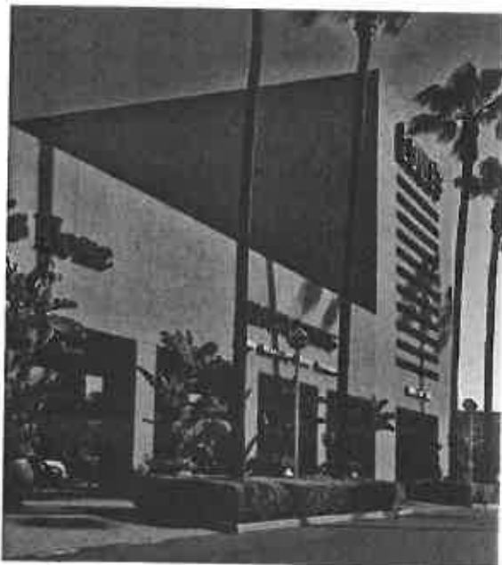
Deep Set Openings
