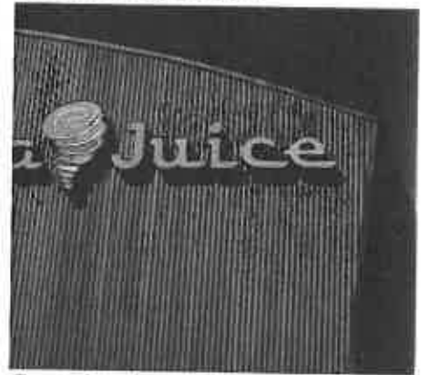
Canted and curved wall with vertical metal siding
