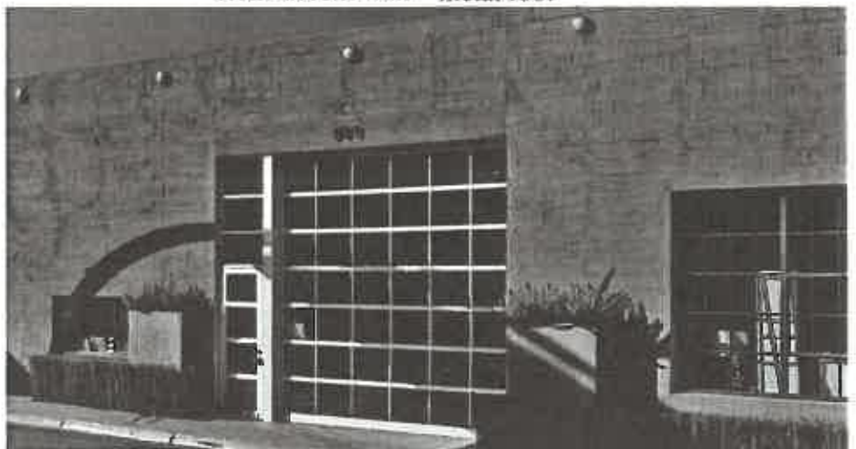
Shot blasted precision concrete block
