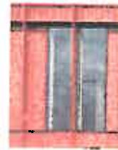
④ Powder coated metal window frames, various colours
