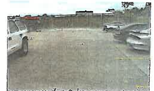
Porous pavements allow water to infiltrate to a soil layer below the surface.
