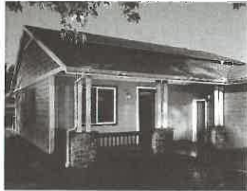
Solar panel placement on front roof elevation
