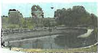
Adaptive measures such as liners, a concrete basin, and overhead wire grid can make extended detention strategies less attractive to hazardous wildlife.
