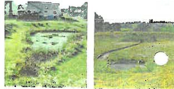
Extended detention basins are frequently used to serve both water quality management and to provide amenities. These basins hold water and would not be appropriate within an AIA because of the open water.
