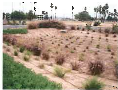
Infiltration Basin (Source: SoCal LID Manual)
