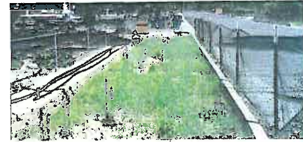
Small bioretention facilities that provide sparse vegetation may be suitable in an aviation environment.
