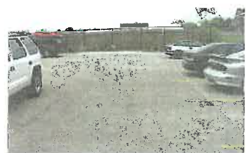
Porous pavements allow water to infiltrate to a soil layer below the surface.
