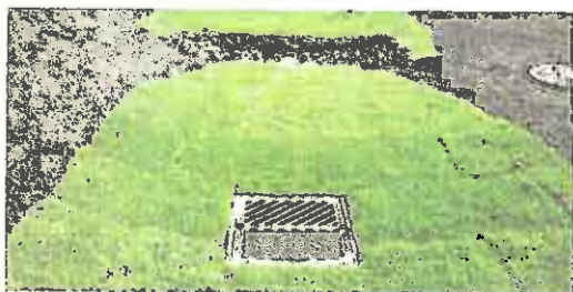
Infiltration trenches detain water for brief periods. This trench at Seattle-Tacoma Airport includes vegetation appropriate for an airport environment.
