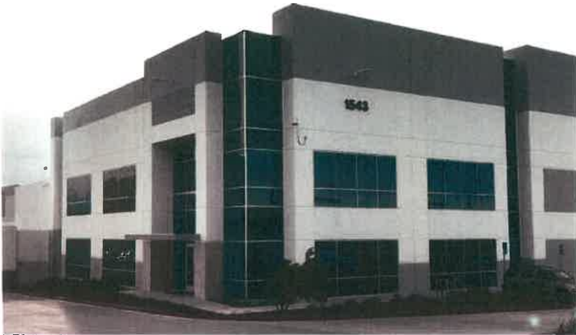
The image above shows the conceptual architectural aesthetic for the Stoneridge Commerce Center.
