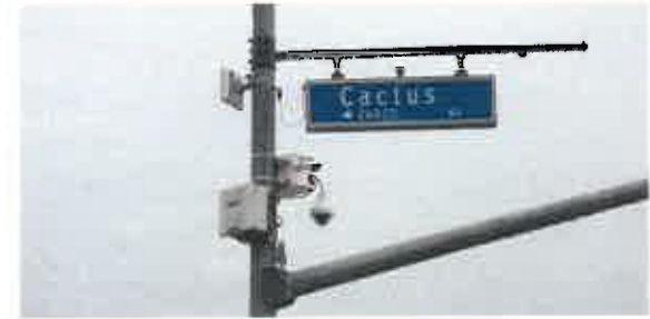
ITS allows the City to monitor different locations strategically and adjust traffic signals to improve flow.
