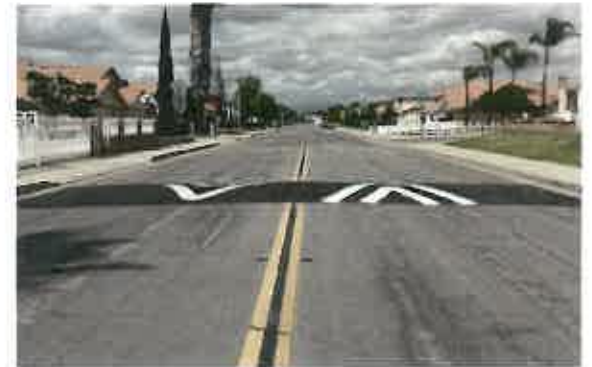
Speed humps are a common traffic calming measure in residential areas.
