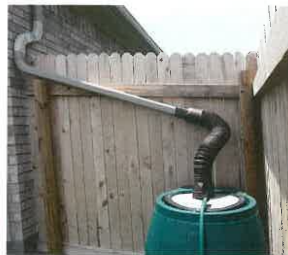
Rainwater harvesting can take the form of a greywater system (left) or a low-tech barrel in one's backyard that stores rain for a future dry day (above).
