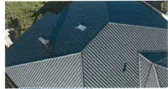
Metal roofs can be a safer decision in wildfire prone areas than other roofing materials.
