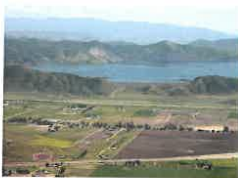
View of Saddle Dam of Diamond Valley Lake
