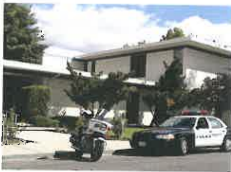
Hemet Police Department Headquarters on Latham Street
