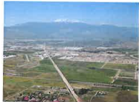
The Hemet/Stetson Channel is one of Hemet's primary stormwater drainage facilities. It runs southwesterly through the City, draining into Salt Creek.
