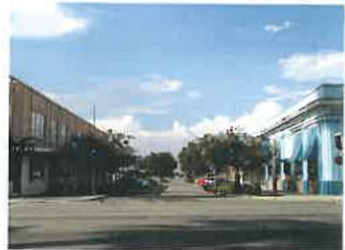
Some of Hemet's unreinforced masonry buildings are located on Harvard Street, north of Florida Avenue, in the City's historic downtown. The City encourages the reinforcement and retention of these historic structures.
