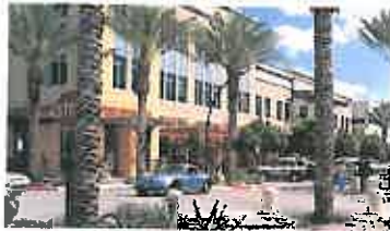
Mixed-use development should support a street-oriented pattern, with buildings sited at or near the sidewalk edge.
