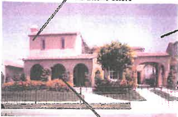
Arches and columns
