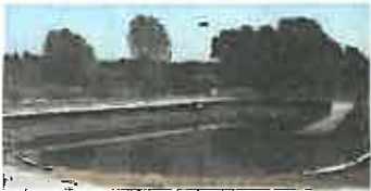
Adaptive measures such as liners, a concrete basin, and overhead wire grid can make extended detention strategies less attractive to hazardous wildlife.
