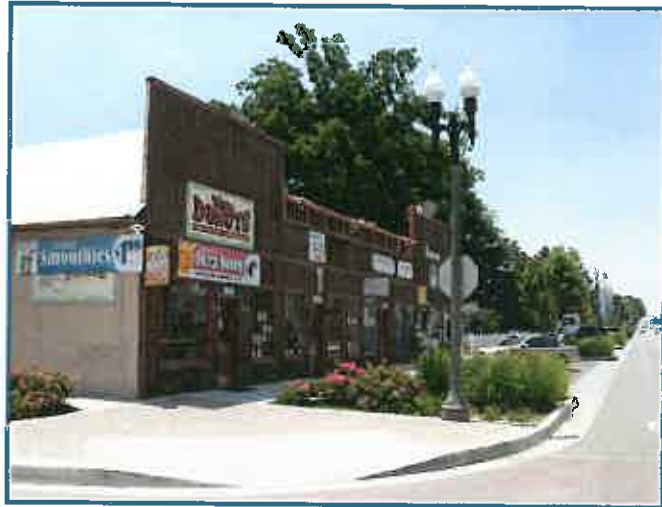
This building on Washington Avenue is believed to be the former A. K. Small & Co. dry goods store, pictured in the Vision chapter as it appeared in 1917.
