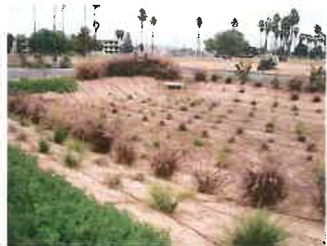
Infiltration Basin (Source: SoCal LID Manual)
