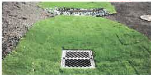
Infiltration trenches detain water for brief periods. This trench at Seattle-Tacoma Airport includes vegetation appropriate for an airport environment.
