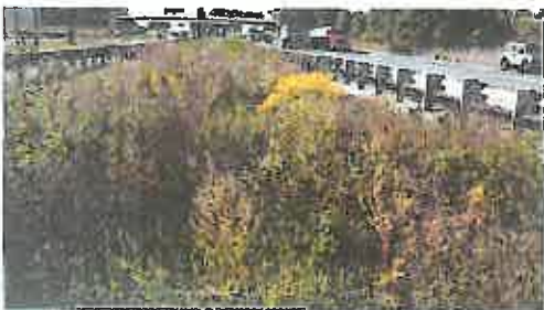
Bioretention facilities can provide food and shelter for potentially hazardous wildlife, but may be suitable with modification.
