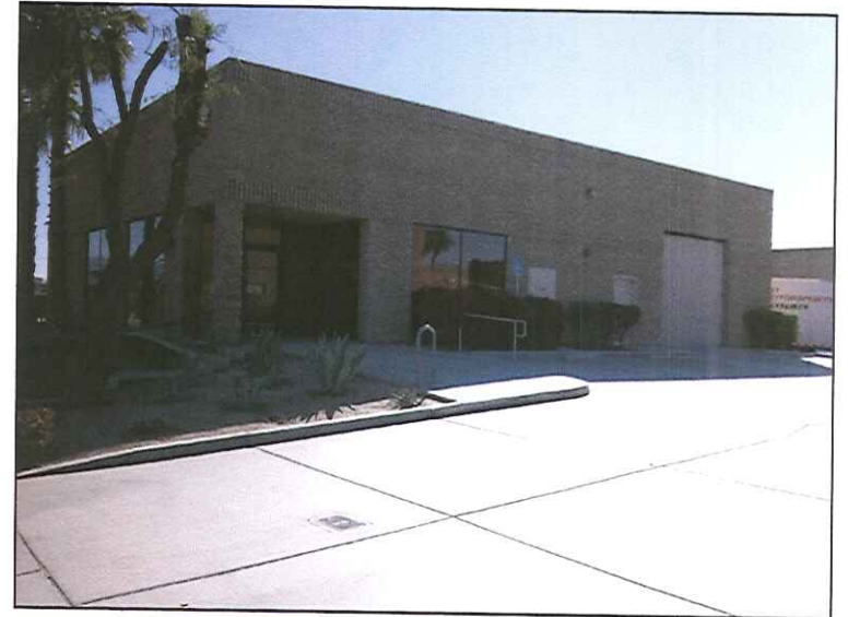
← Photo taken from the intersection of Wildcat Dr & Racoon St (northeast of building), looking southwest.
